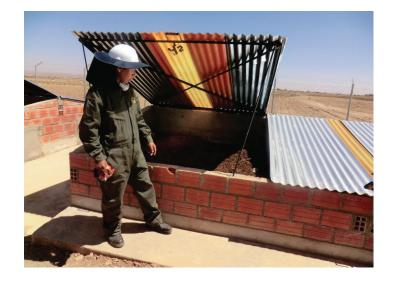
Citations: Hill, G.B., Baldwin, S.A., 2012. Vermicomposting toilets, an alternative to latrine style microbial composting toilets, prove far superior in mass reduction, pathogen destruction, compost quality, and operational cost. Waste Manage. (Oxford) 32 (10), 1811–1820.
